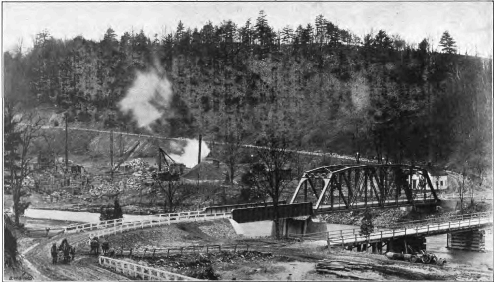
SCHOHARIE RESERVOIR—Looking southwesterly from Road 9, showing the new Schoharie steel highway bridge and the temporary bridge across the Schoharie creek in right foreground with the Riverside quarry in left background. Road 8 can be seen on the far side of the stream.
