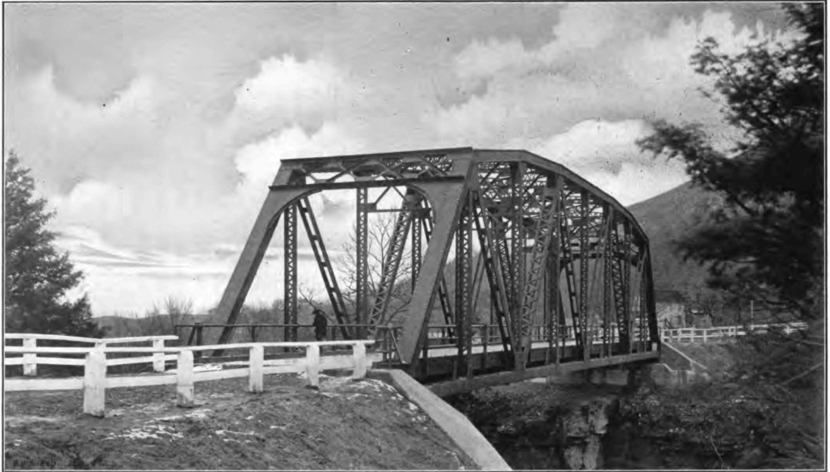
SCHOHARIE RESERVOIR—The Manor Kill bridge looking westerly. Details of the bridge seat on the west abutment can be seen in this view. The floor consists of an 8-inch concrete slab carrying the 2-inch asphalt-block pavement.
