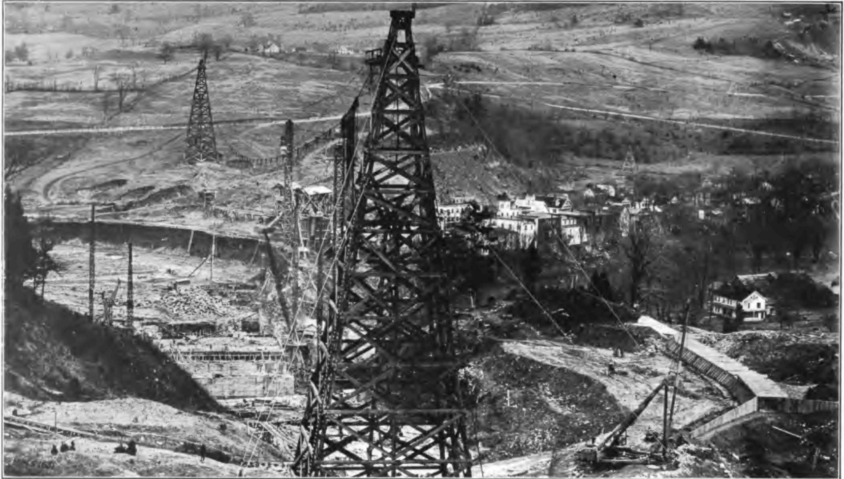
SCHOHARIE RESERVOIR—General view of construction work on the Gilboa dam, looking easterly. The masonry placed in the dam is shown to the left of the cableway tower in foreground with excavation for the spillway channel in progress beyond. The full length of the stone tramway is shown in this view. In right foreground are the Steen Kill dike and temporary flume. In the background Road 1 and the temporary road can be seen with the crusher plant and quarry on Stevens mountain at extreme right.
