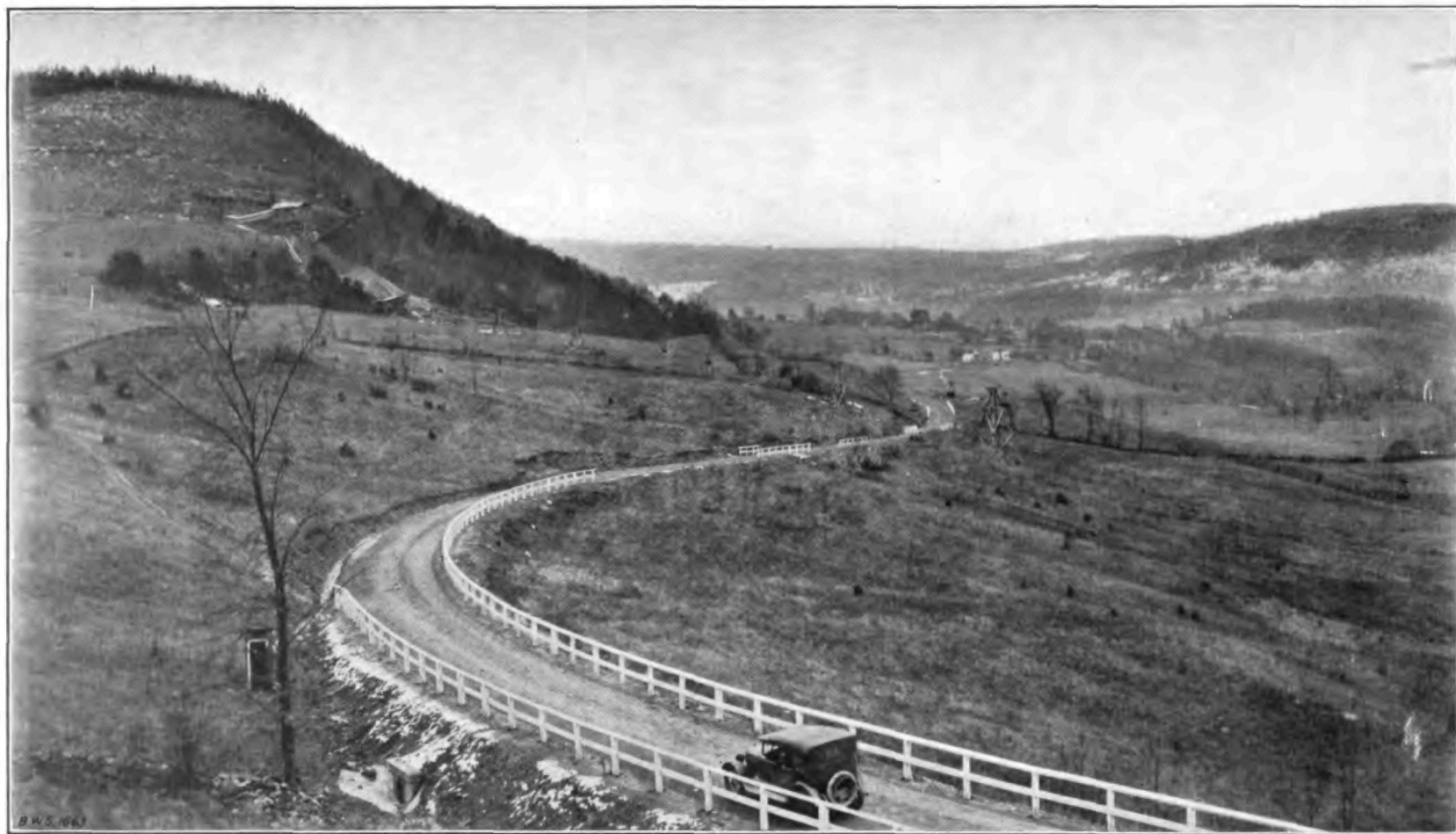
SCHOHARIE RESERVOIR--Looking easterly along Road 1. In left background can be seen the Stevens Mountain quarry and crusher plant, and leading therefrom is the tramway for conveying crushed stone to the site of the Gilboa dam.
