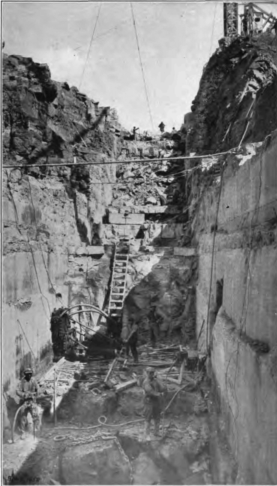
SCHOHARIE RESERVOIR—Excavation for the Gilboa dam, looking easterly along the cut-off trench. The bottom of the cut-off is at Elevation 949. |
