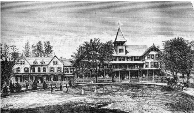
The Cave House and the Pavilion Hotel (right).
