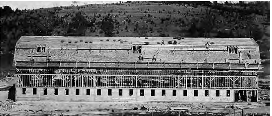
The beams and some of the 2 x 4s were in place for the second-floor walls when a windstorm came through on March 23, 1923. By late spring, the mess was cleaned up, more 2 x 4s and the roof were put in place, and shingles were being placed on both the west side (below) and east side (bottom). The east side had entrances for two bridges to allow hay wagons into the hay mow.
