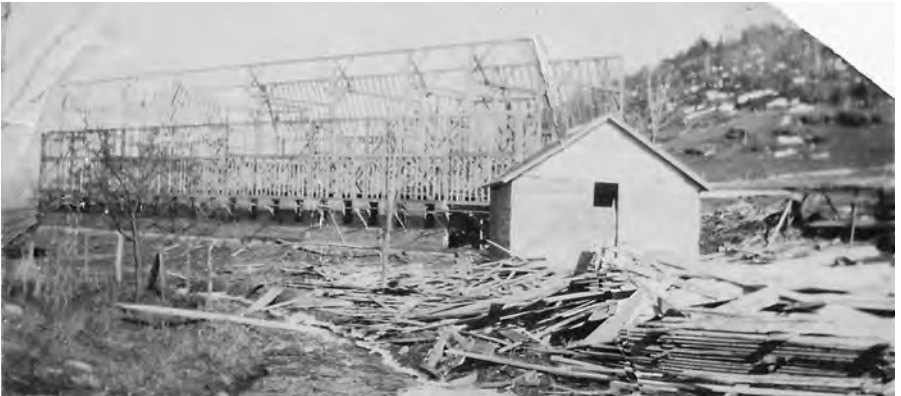
The beams and some of the 2 x 4s were in place for the second-floor walls when a windstorm came through on March 23, 1923. By late spring, the mess was cleaned up, more 2 x 4s and the roof were put in place, and shingles were being placed on both the west side (below) and east side (bottom). The east side had entrances for two bridges to allow hay wagons into the hay mow.
