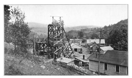
The infrastructure above shaft 4 was duplicated above each of the shafts. The tall structure is the head frame above the shaft, used to transport sandhogs to the work areas, to supply fresh air to the workers, and to remove displaced dirt from the tunnel. The other buildings were used for housing and management. 16th Annual Report of the Board of Water Supply (1/1/1922)
