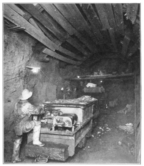
Muck from the tunnel was loaded into cars and hauled to shaft 6 for removal. The platform in the background is used to place timbering. 16th Annual Report of the Board of Water Supply (1/1/1922)
