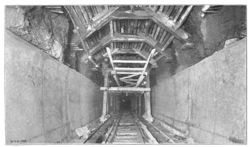
Looking to the south between shafts 5 and 6, showing the completed sidewalls and permanent timbering. 17th Annual Report of the Board of Water Supply (1/11/1923)
