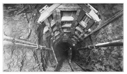
A completely dug-out and reinforced section of the tunnel below shaft 6 being prepared for concrete. 16th Annual Report of the Board of Water Supply (1/1/1922)
