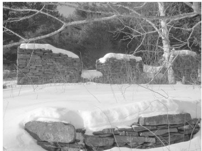
The foundation and laid stone walls of the livery stable serving the stage coaches on the branch line of the Catskill Turnpike.
