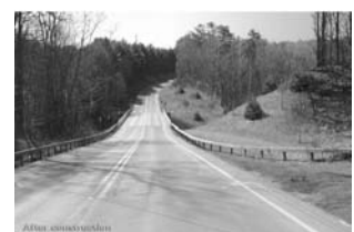
Road after reconstruction
