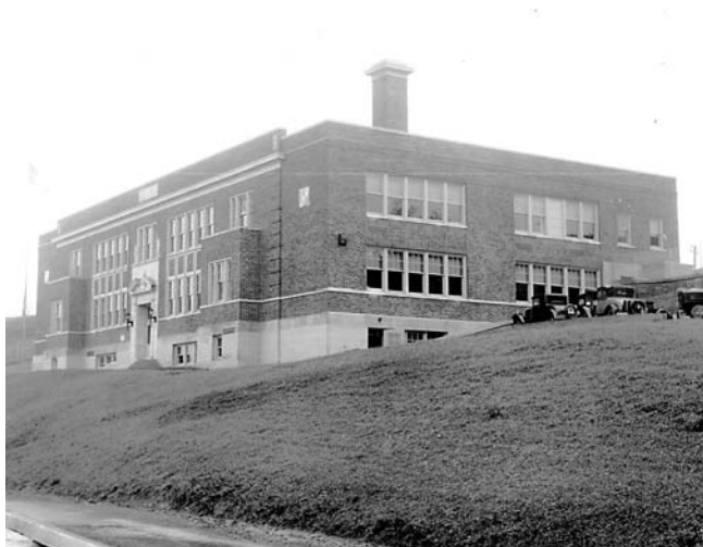
The new Gilboa-Conesville Central School, photo courtesy of Joan Hess Mullen
